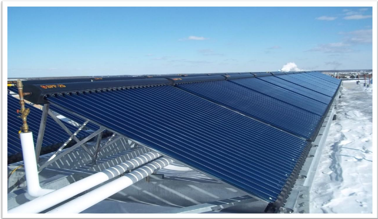
Solar panels on the roof of the EHS Building
